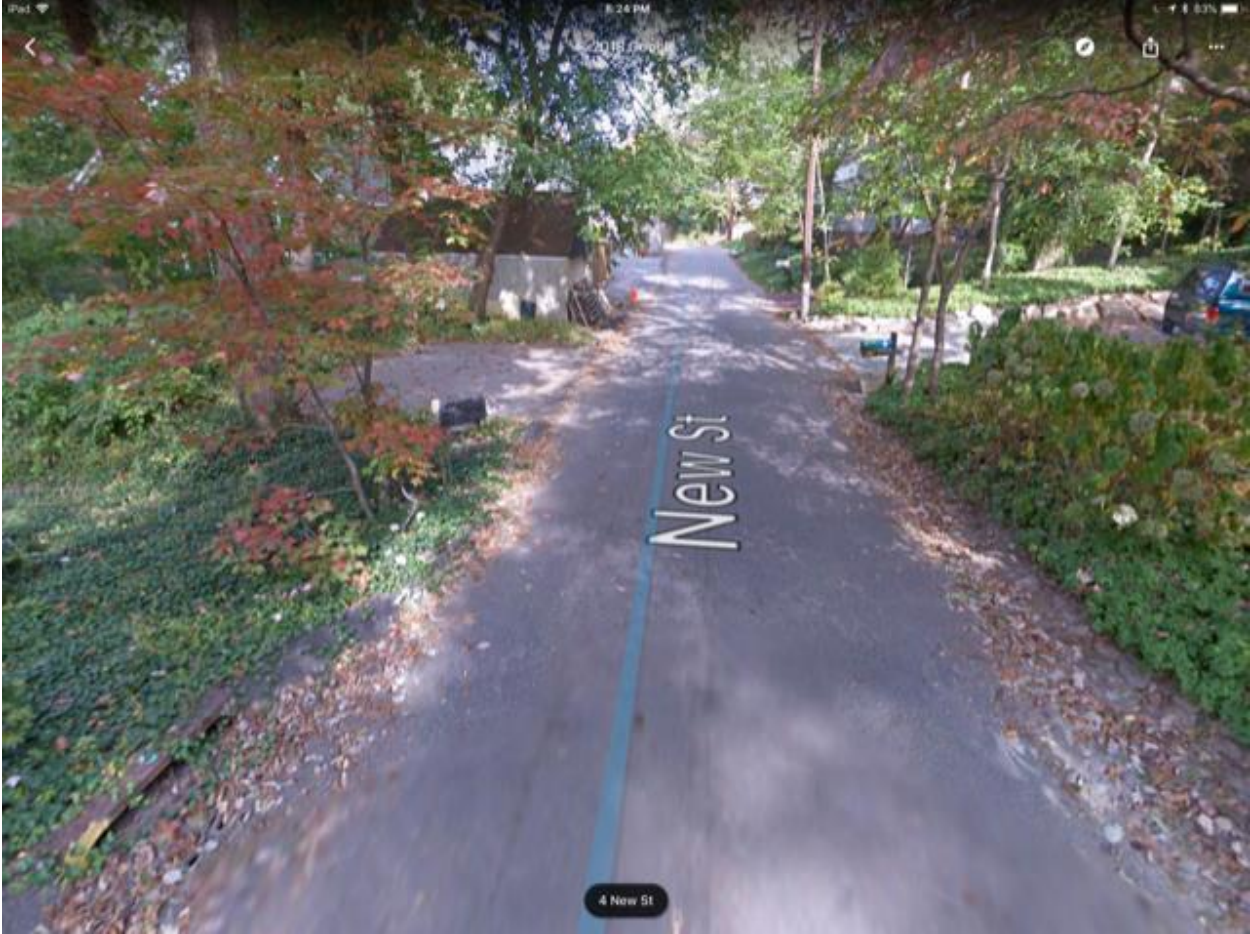
New Street with drain 21 on left and 22 in background.
