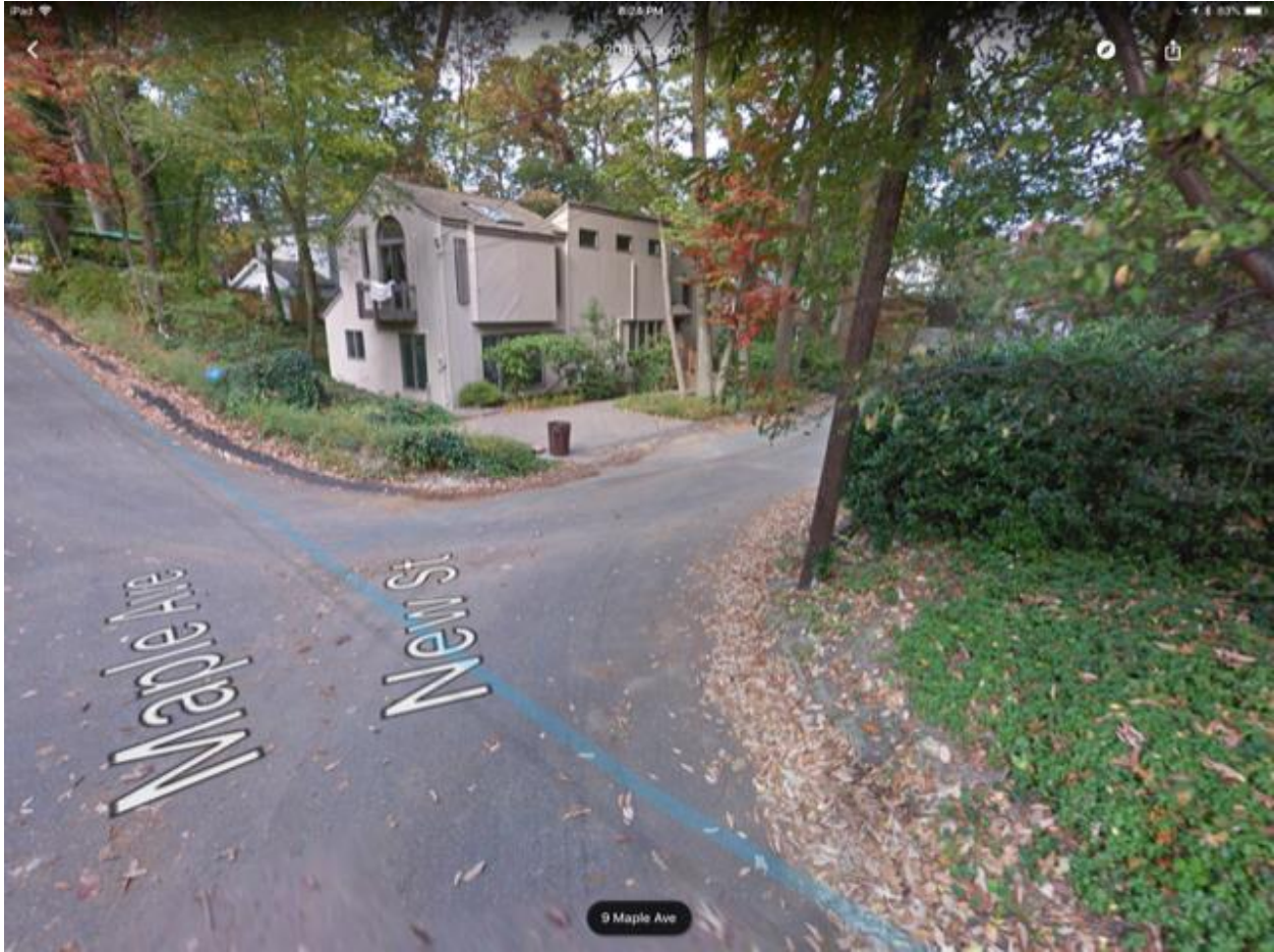
Intersection of New Street and Maple Avenue. Note: significant evidence of runoff and erosion and debris in roadway coming from both the east and west sides of Maple Avenue.
